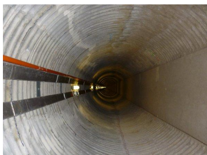
Inside Burdekin Falls Dam
